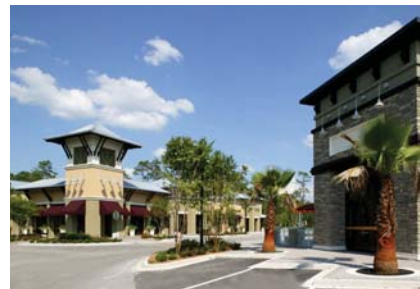
Hard hats off to the following project team leaders for a job well done: Jeff Kleffman, AWC Project Manager; Mike Luke, AWC Superintendent; Tim Miller, Project Architect; Becky Mariotti, Gate Land Development.
