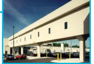
Vistakon Injection Molding Renovation, 1st Project for Vistakon
