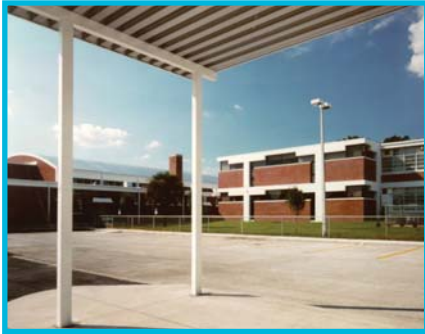
James Weldon Johnson Renovation, 1st Project for Duval County Public Schools
