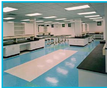
Florida Department of Health, Central Lab Addition & Renovation, 1st Project for FDOH
